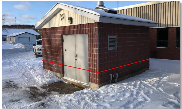
Figure 4.6: Exterior of Magnolia Avenue Well House, with predicted 2100 1:100 flood elevation of 21.61m shown.
