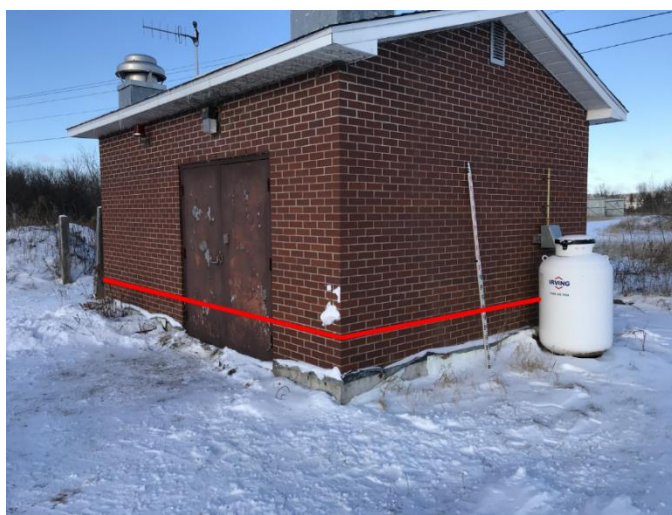
Figure 4.1: Exterior of Stewart Avenue Lift Station, with predicted 2100 1:100 flood elevation of 18.86m.
