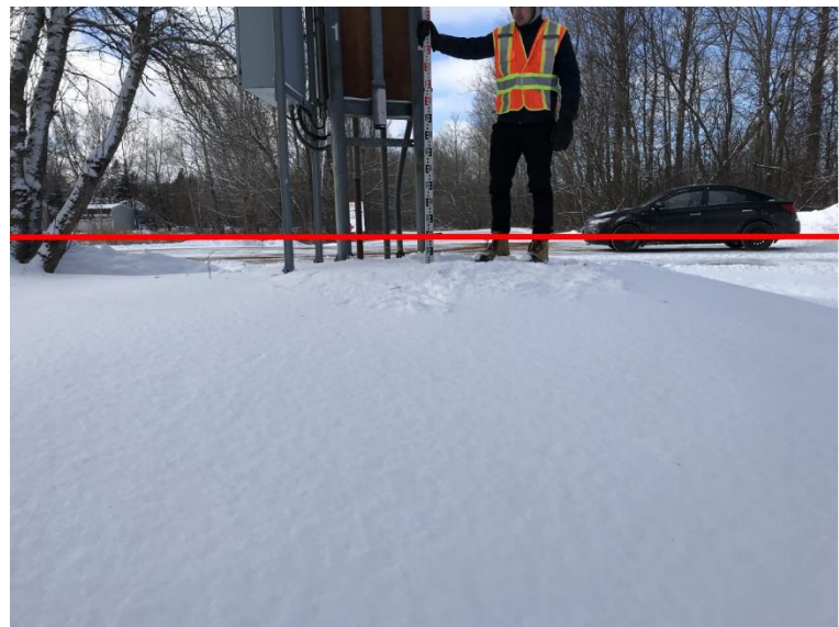
Figure 4.4: Willow Court Lift Station, with predicted 2100 1:100 flood elevation of 22.19m.
