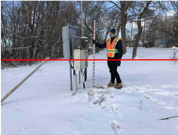
Figure 4.3: Main Street Lift Station, with predicted 2100 1:100 flood elevation of 22.91m.
