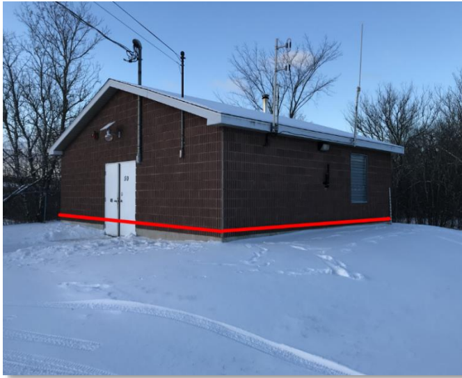
Figure 4.5: Exterior of Jonah Court Well House, with predicted 2100 1:100 flood elevation of 25.20m shown.
